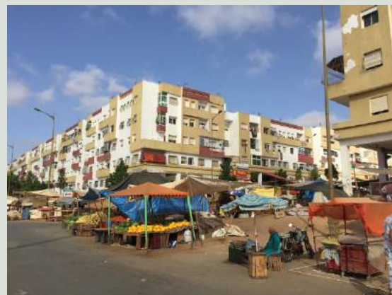
The city of Tamasna, in the rural region of Sidi Yahya Zaer, 20km from Rabat, has failed to deliver what it promised, including supporting social infrastructure
